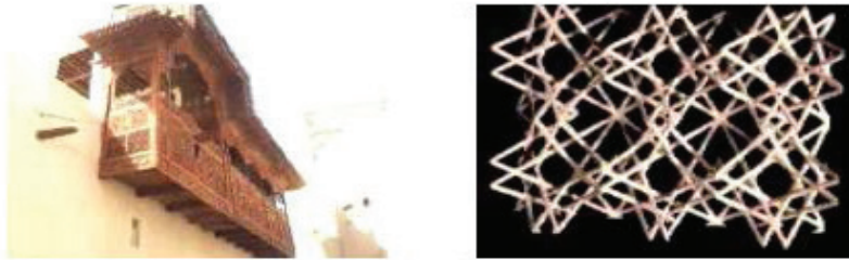
Figure 15. From left: a traditional Mashrabiya, a 3d printed Mashrabiya model by the SLS technology (Almerbati and Headley, 2016)
